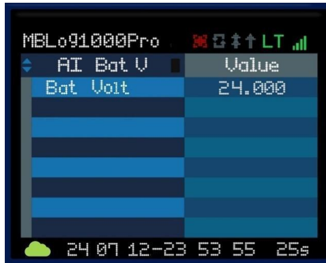
Figure-4.11: Measured battery voltage value
