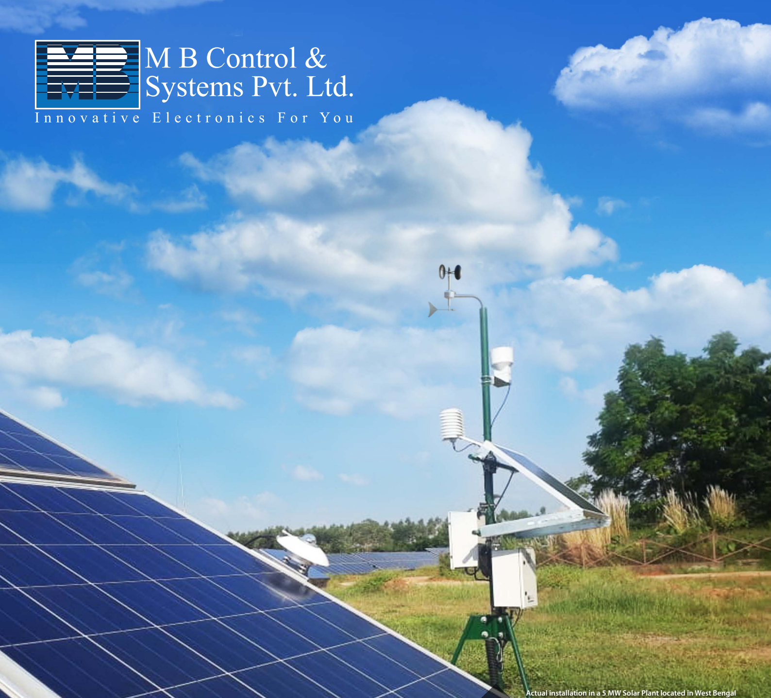
Actual installation in a 5 MW Solar Plant located in West Bengal
